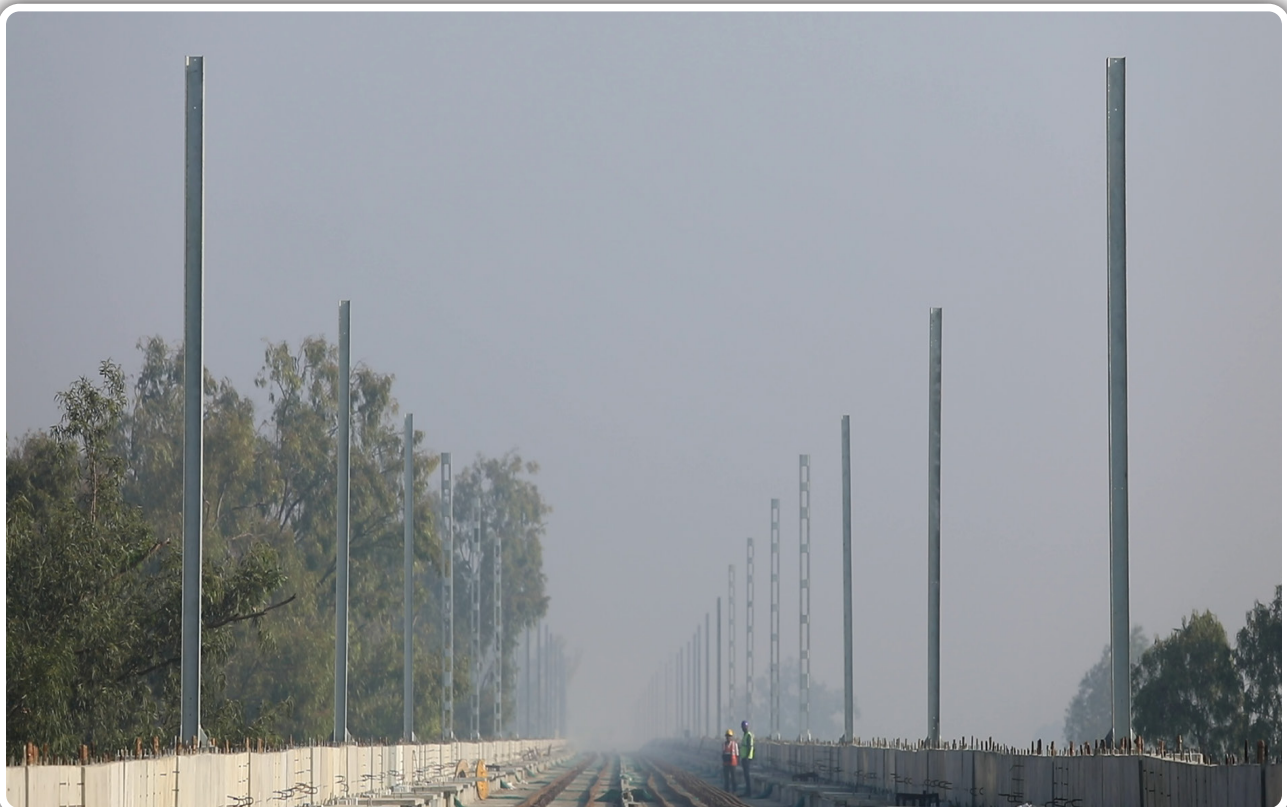
OHE Masts installation
