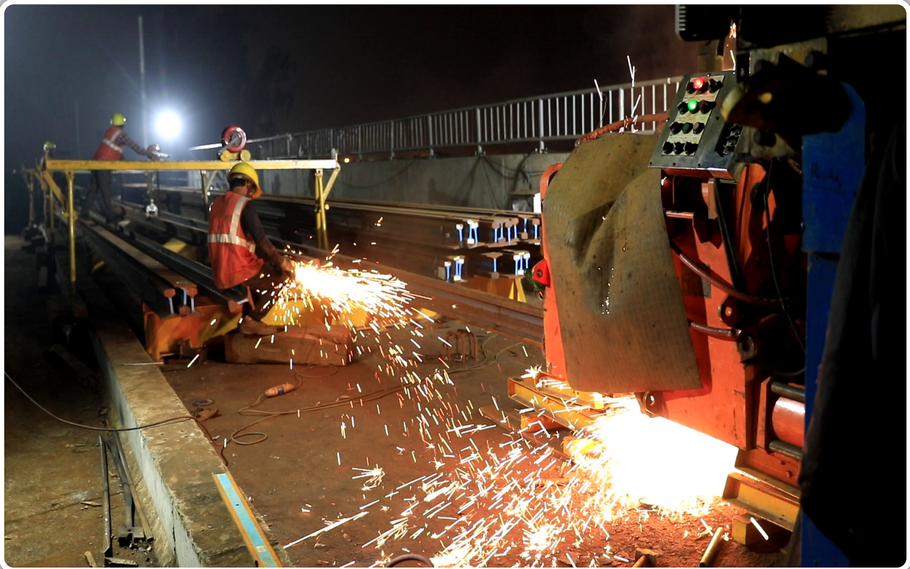
Flash Butt Welding of Rails on Viaduct
