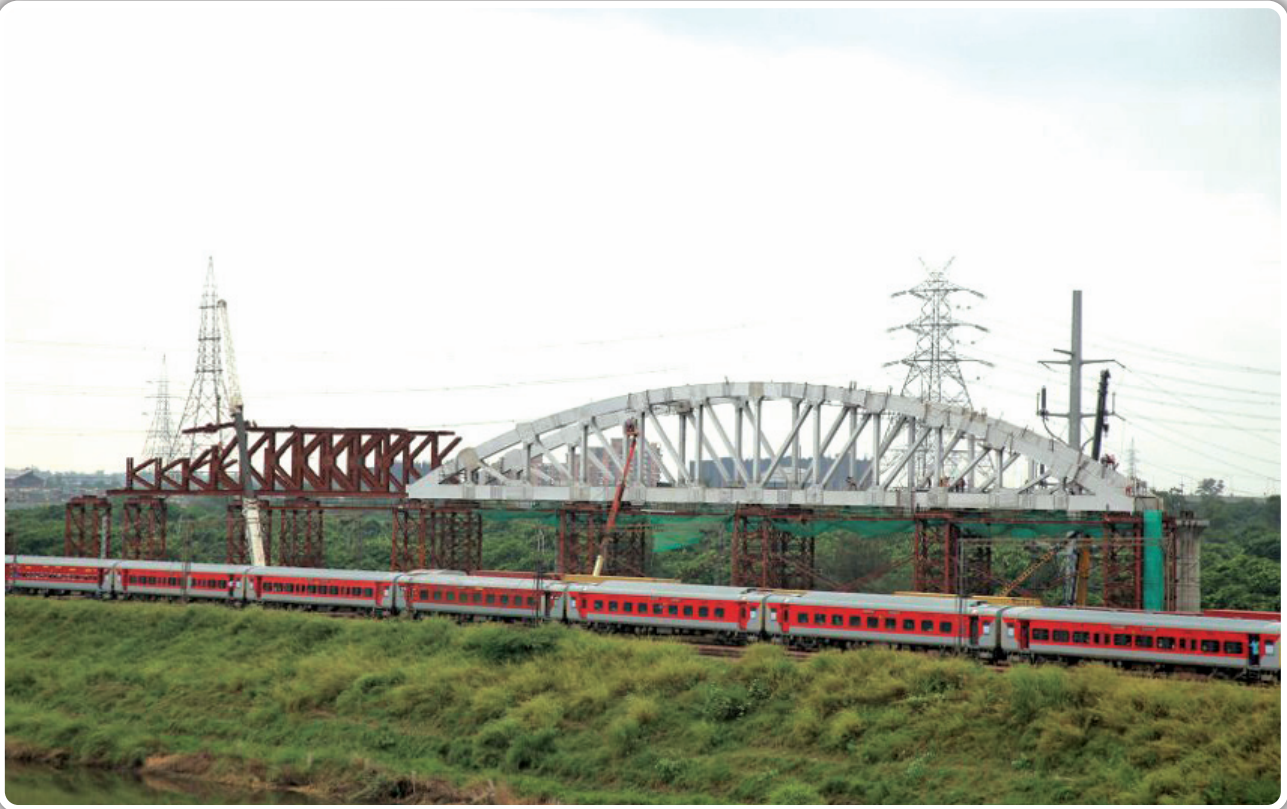
Assembly of a special span at a railway crossing near Ghaziabad
