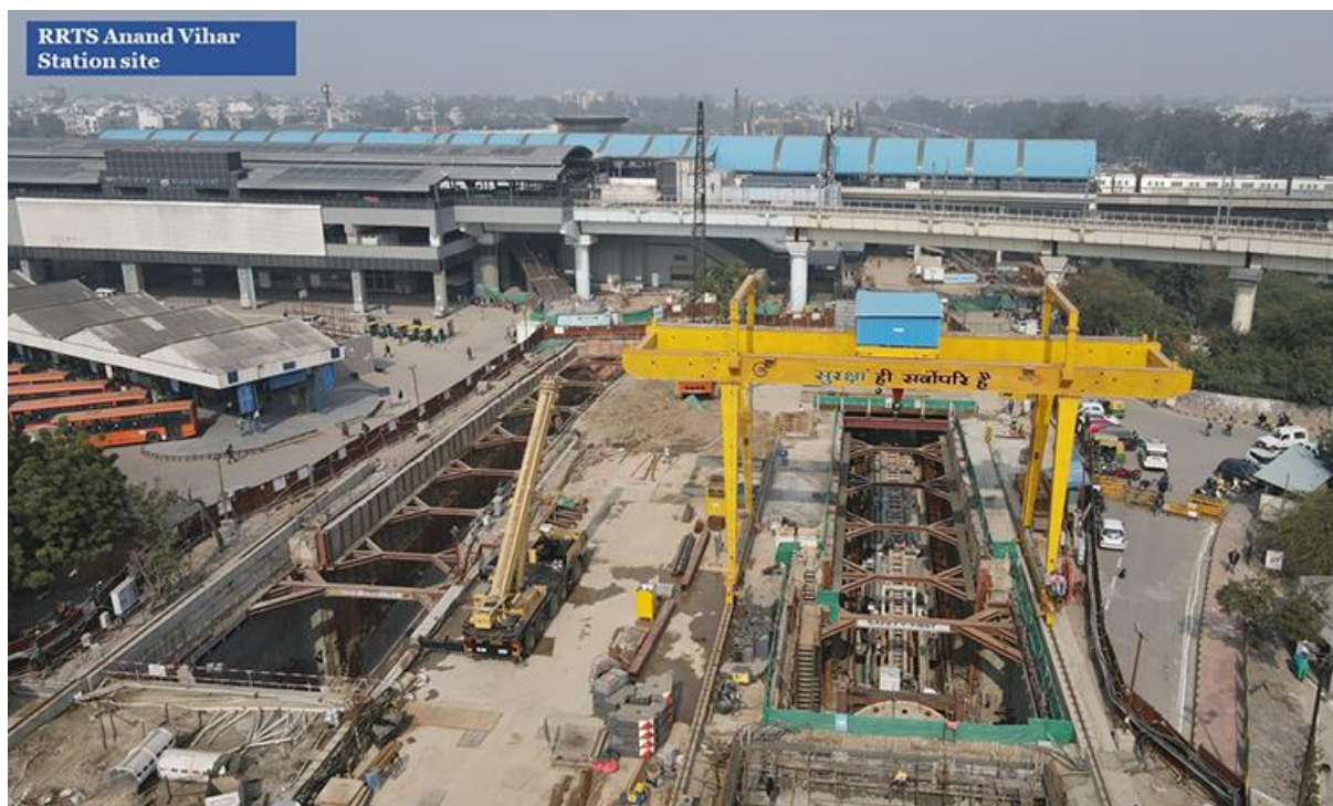
Credit: NCRTC – Construction work at the RRTS Anand Vihar station site.
