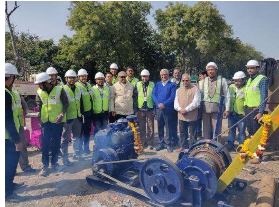
Geotechnical investigation works – in progress
