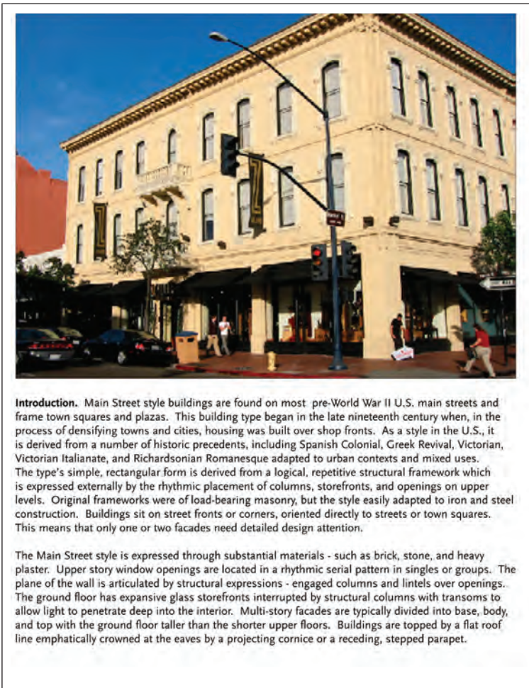
Figure 41: Aspects related to architectural standards covered in FBC for city of Whittier (City of Whittier)
