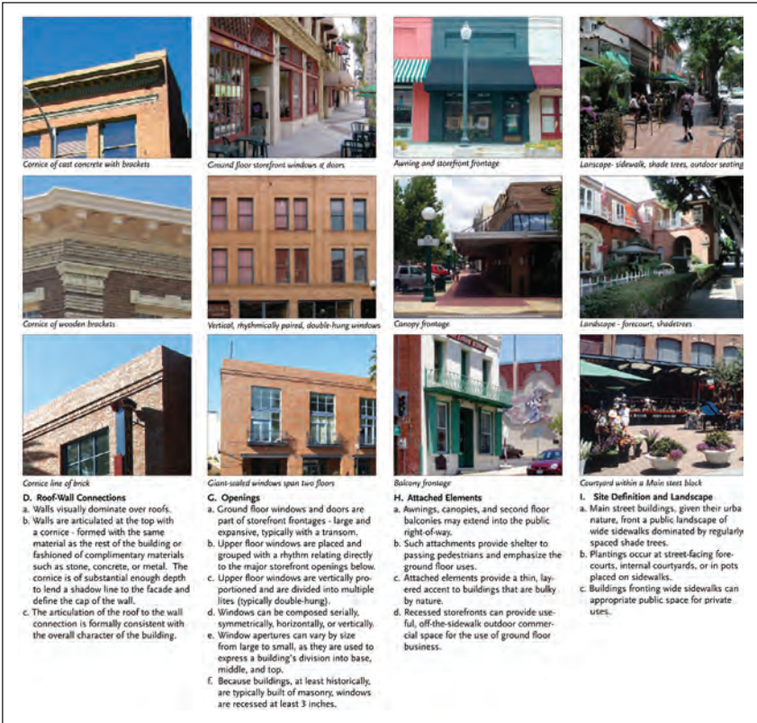
Figure 43: Aspects related to architectural standards covered in FBC for city of Whittier (City of Whittier)
