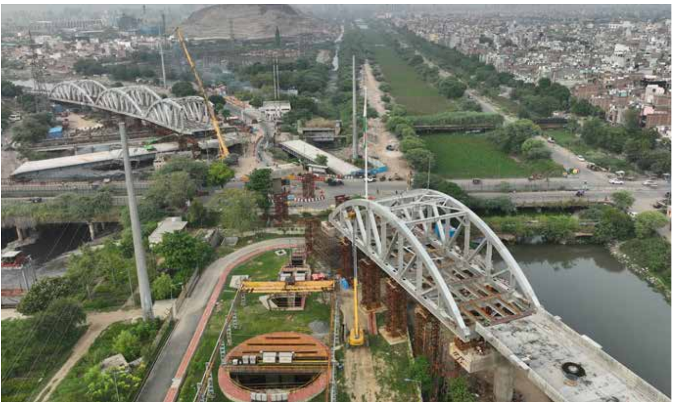
6 giant special steel spans being installed at Kondali, Delhi to cross Ghazipur Drain
