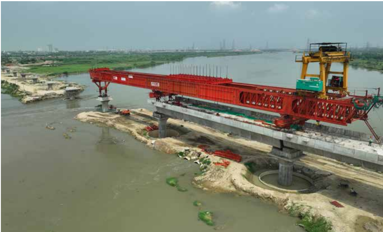
Construction of viaduct for RRTS to cross over river Yamuna approaches completion
