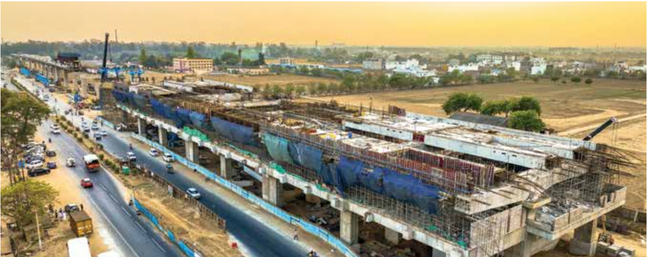
Construction work in Meerut progressing swiftly and nearing completion
