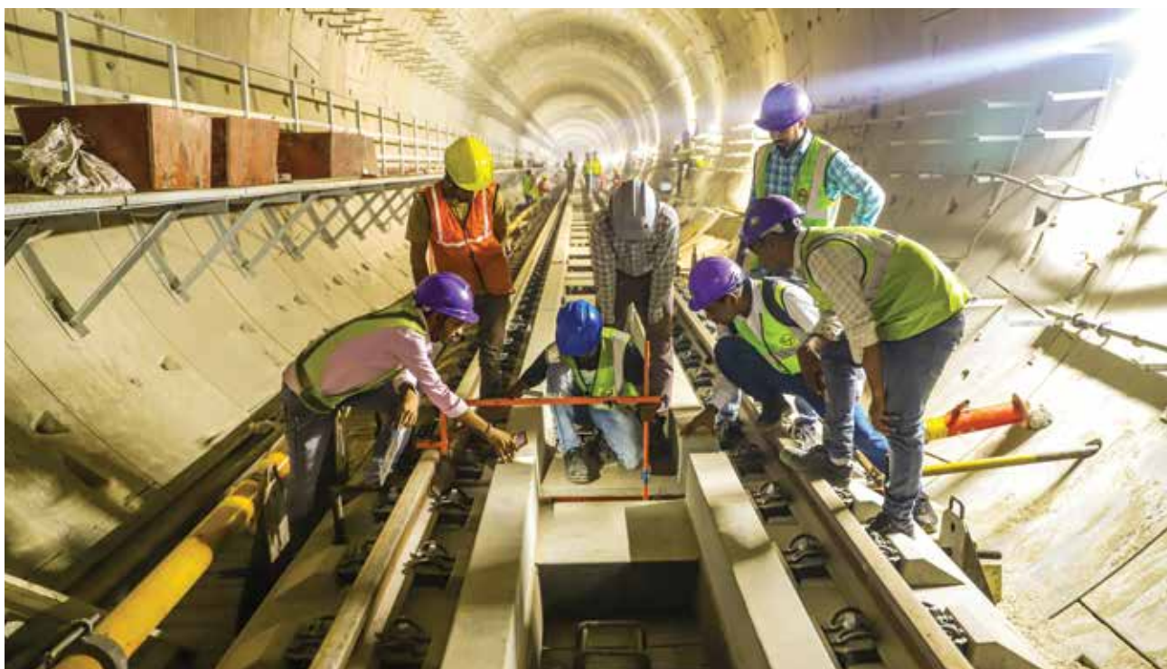
Work on the corridor progressing round-the clock = for timely completion
