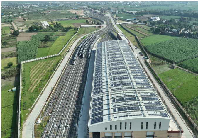
Solar-powered depot for a sustainable future
