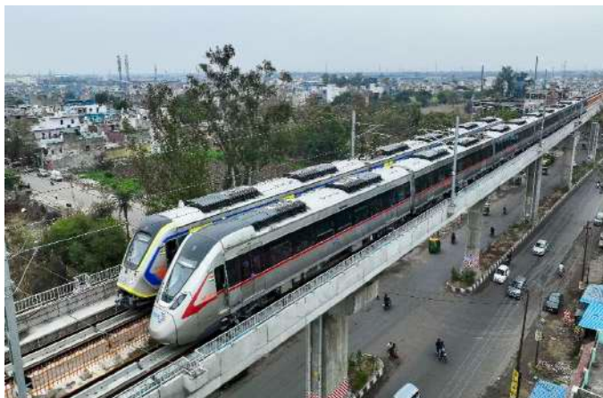
Namu Bharat and Meerut Metro trains traversing on the Viaduct
